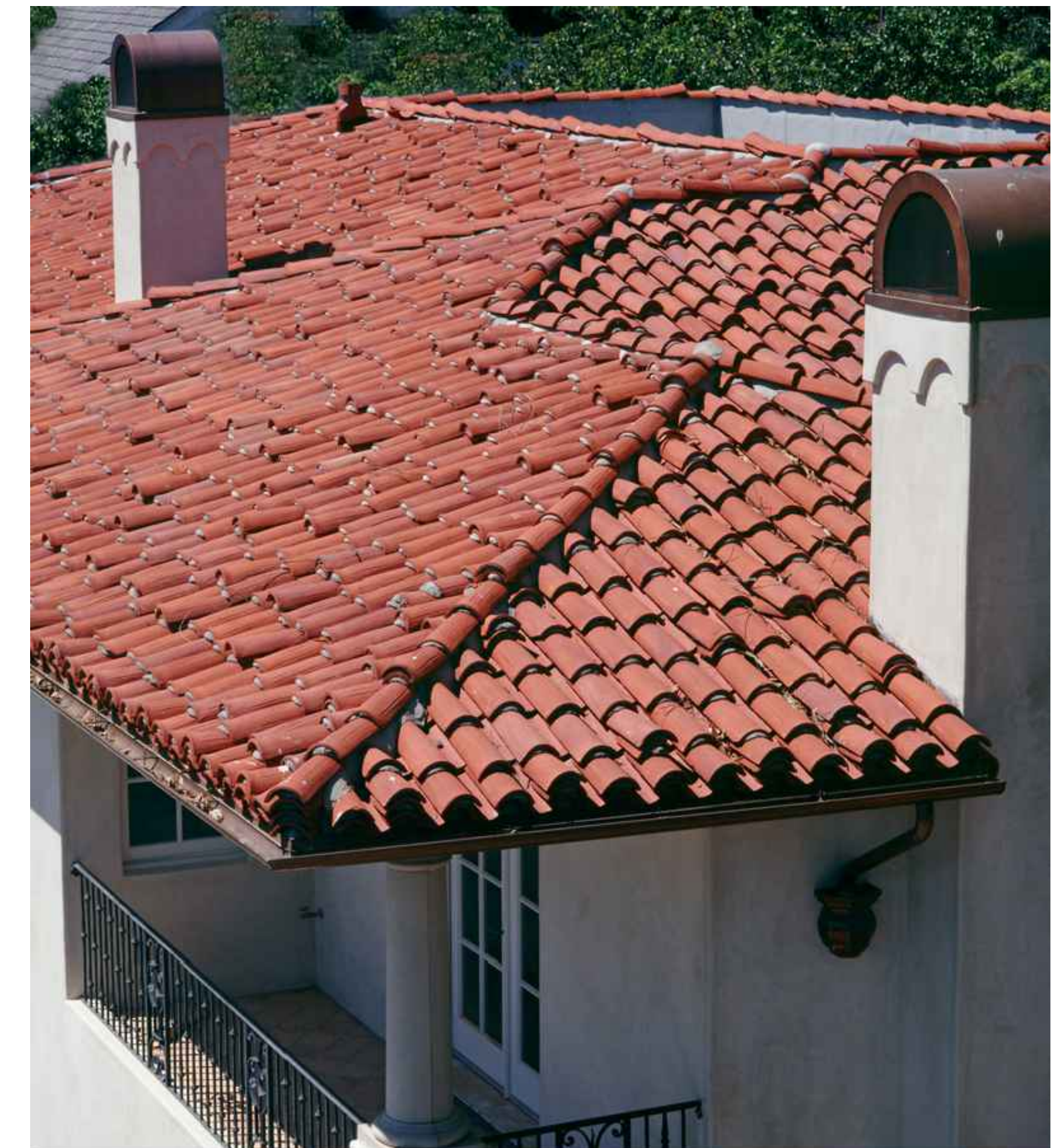
HIGH BARREL STAGGERED CLAY TILE ROOF
